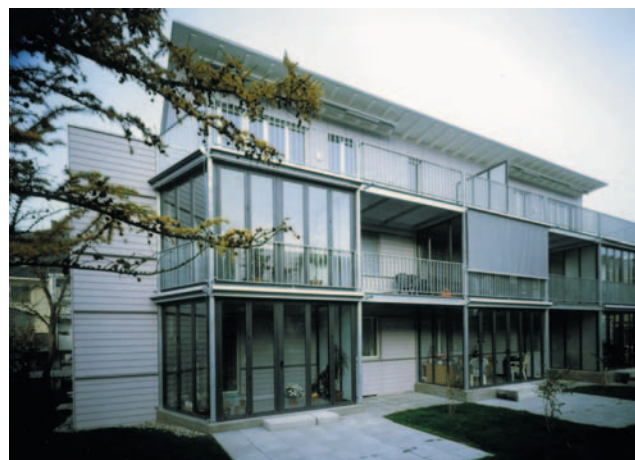
Fig. 4.1-3: Retrofit Demonstration Building Therwil (CH): after renovation and added penthouse, 1/4 of original energy demand for heating and hot water (~ 50 kWh/m 2 )
