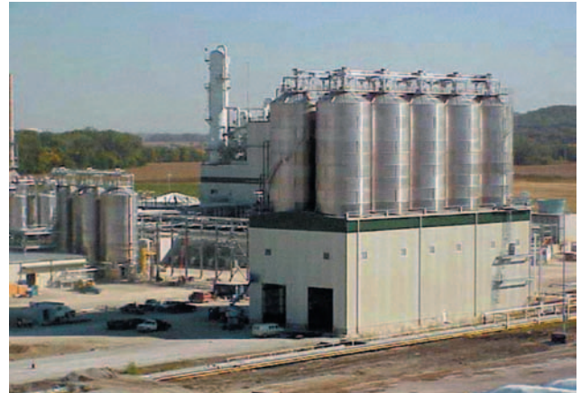
Fig. 4.4-2: Production plant for polyactide from starch (Blai, Nebraska, USA), 140 000 t/a, 10 years development
